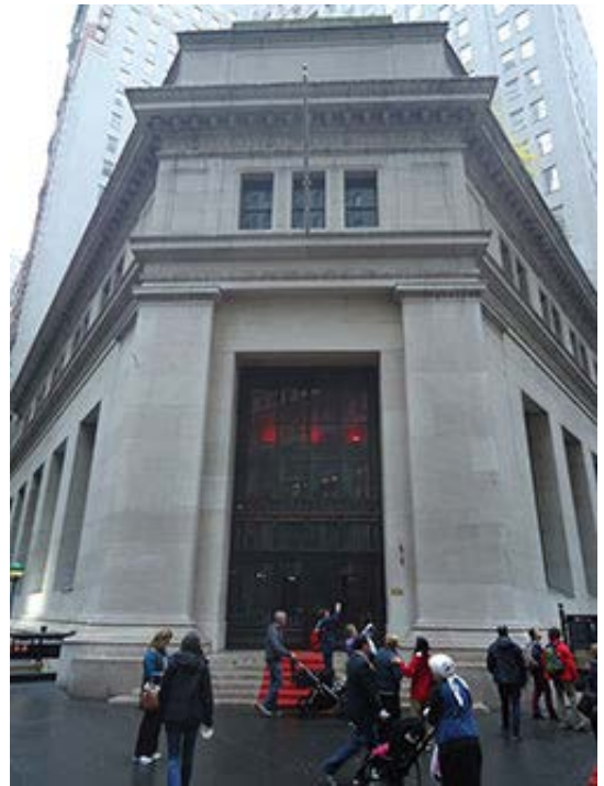
23 Wall Street, the former JPMorgan building in New York now owned by China Sonangol
